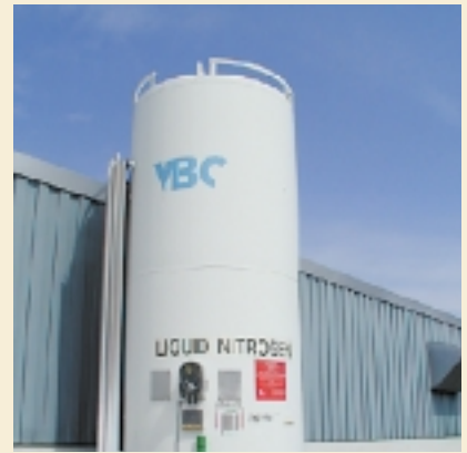
Both portable dewars and bulk tank-fed systems can be used with nitrogen dosing systems. Because of their size, portable dewars (left) must be refilled regularly, but bulk tank systems (right) do not.
