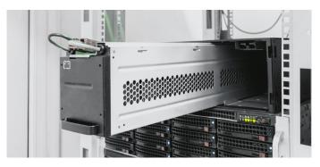
**Uninterruptible Power Supply**Vital for data protection, the UPS provides a dependable power source to mitigate data loss and maintain continuous operation of critical systems during power interruptions
