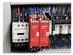
Redundant safety loop Secondary safety system provides full back up to primary safety circuit
