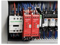
**Redundant safety loop** Secondary safety system provides full back up to primary safety circuit
